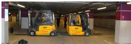
Fig. 2. Slab loaded with forklifts.
