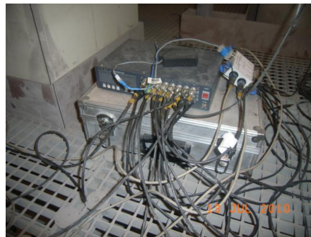
Fig.2 Measuring equipment used in the measurements - multi-channel recorder
