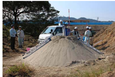
Fig.1 Sand embankment used for injection test.
